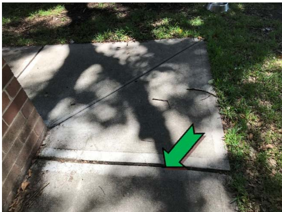
Photo 3. Exterior, throughout, ground, expansion joint – non asbestos-containing construction joint mastic.
