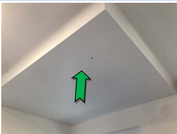
Photo 5. Interior, disabled toilets, boxing – non asbestos-containing fibre cement sheeting.
