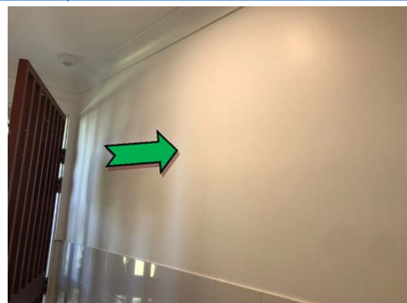
Photo 6. Interior, ladies toilet, east wall – non asbestos-containing fibre cement sheeting.
